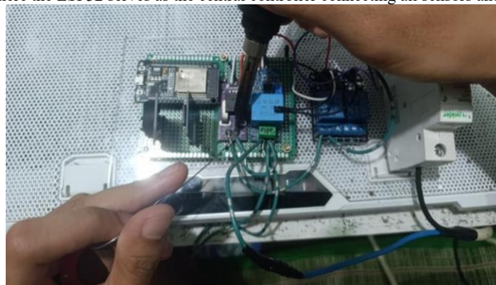
Fig. 5: Installation of All Components
